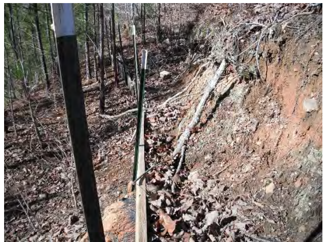
Due to the steepness of the slope, erosion on the face of the slope was observed during the inspection. No soils were observed to have migrated offsite.
