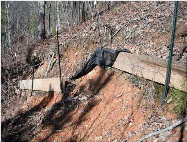
The BMPs repaired in March of 2015 were observed to be in place and in good condition.
