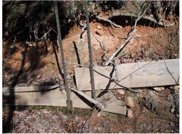
The t-posts located behind the wooden board helps to keep the board in place and helps limit erosion.
